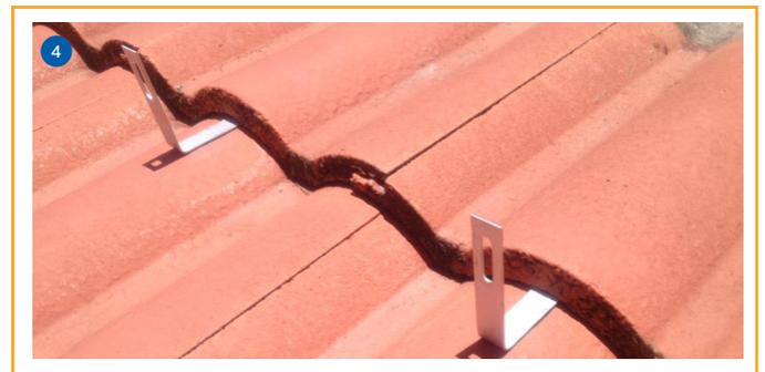
Tip: Before screwing bracket, tap bracket with a hammer to help mould around the tile and against the timber batten, this will help when screwing bracket to batten.
